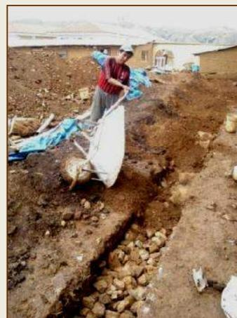
RELLENO FINAL DE ZANJAS DE DESAGUE CON MATERIAL PROPIO
