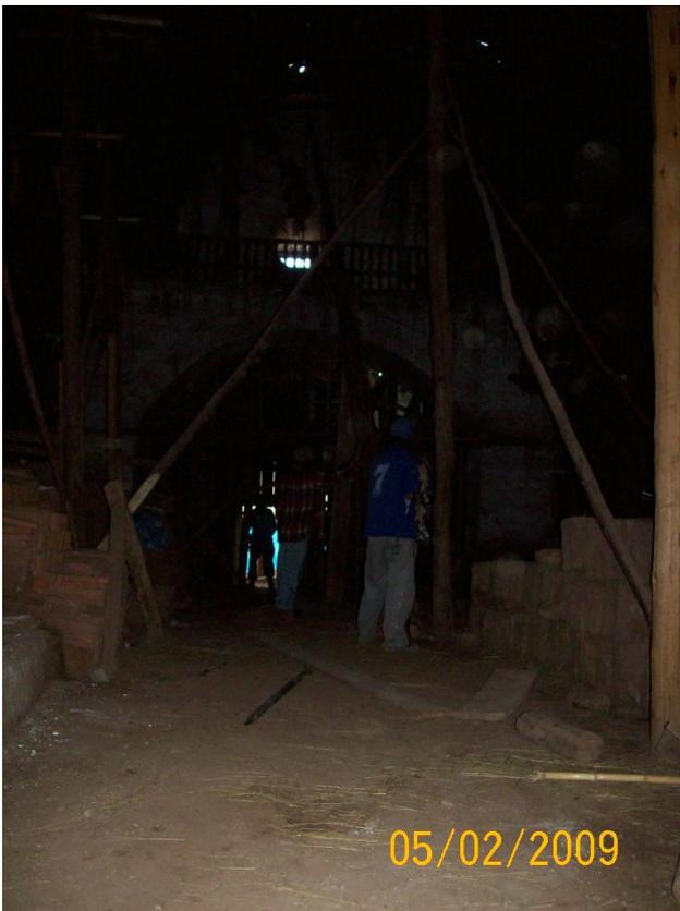
APUNTALAMIENTO DEL ASTIAL DEL MURO DE PIES, CON PUNTAL Y TABLERO TIPO DOBLE.
